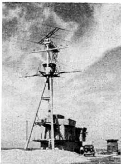
Rotary beam—U.S. Navy style. The aerial system at JA2KW looks very much as though someone has lost part of a battleship!
